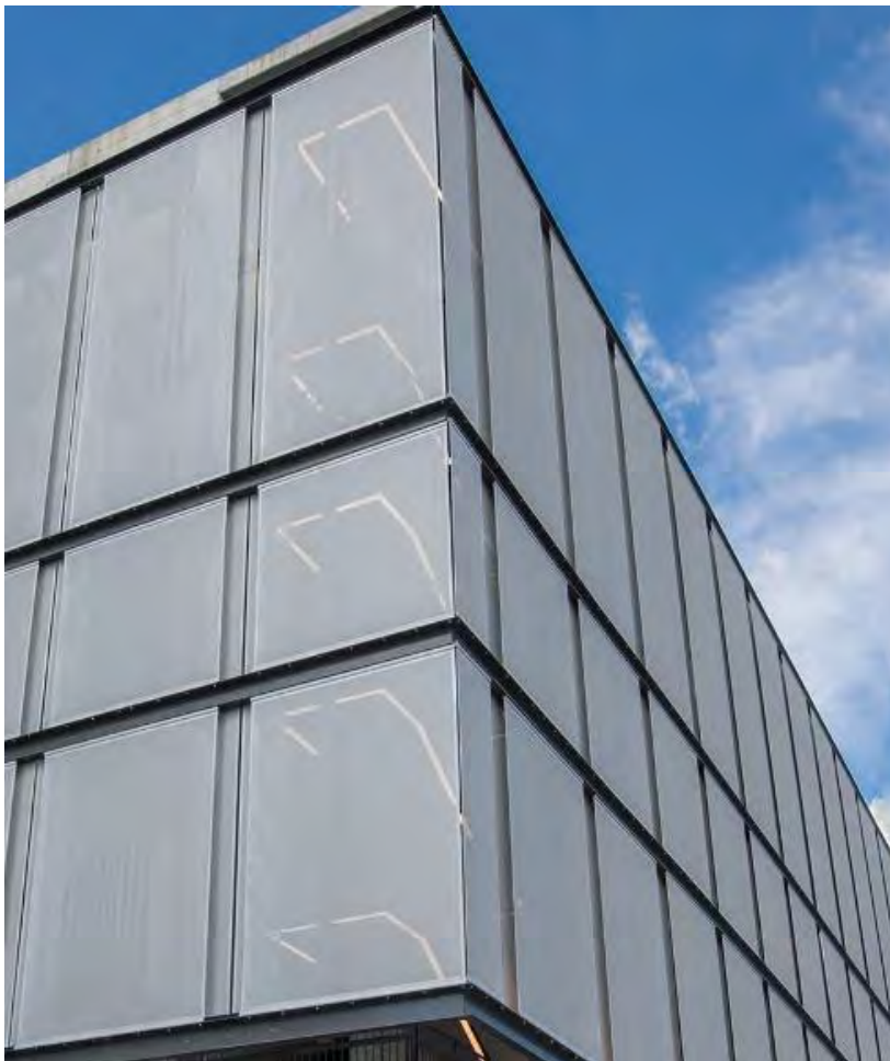
Examples of Buildings with Aluminum Frame and coated PES and PTFE material.
